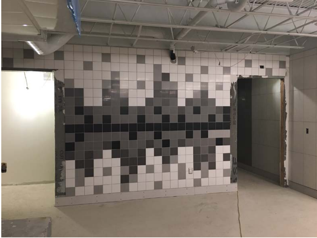
Ceramic tile work at the High School Locker Rooms.
