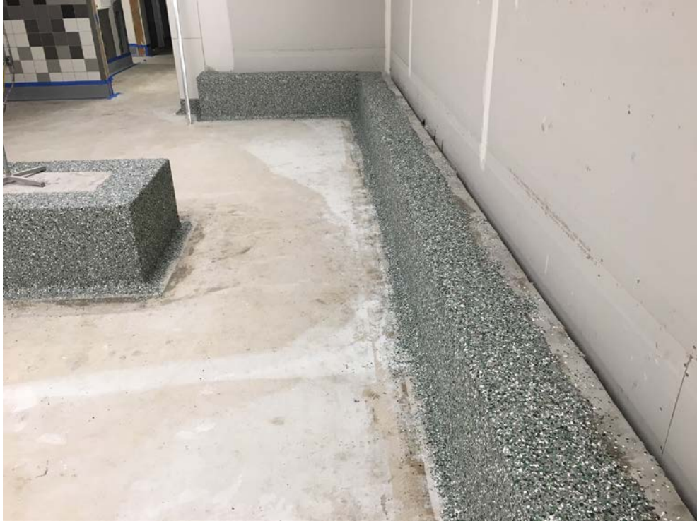
Epoxy floor coating installed on HS Locker Room locker bases.
