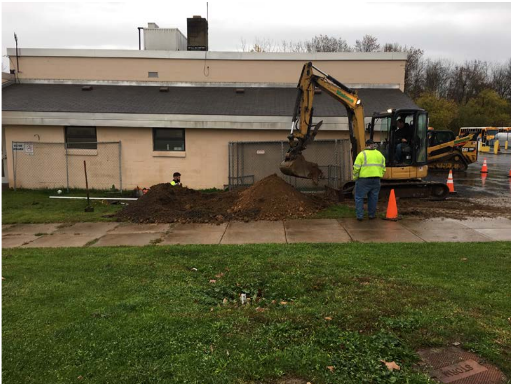
Excavation for new force main pipe behind the Bus Garage.
