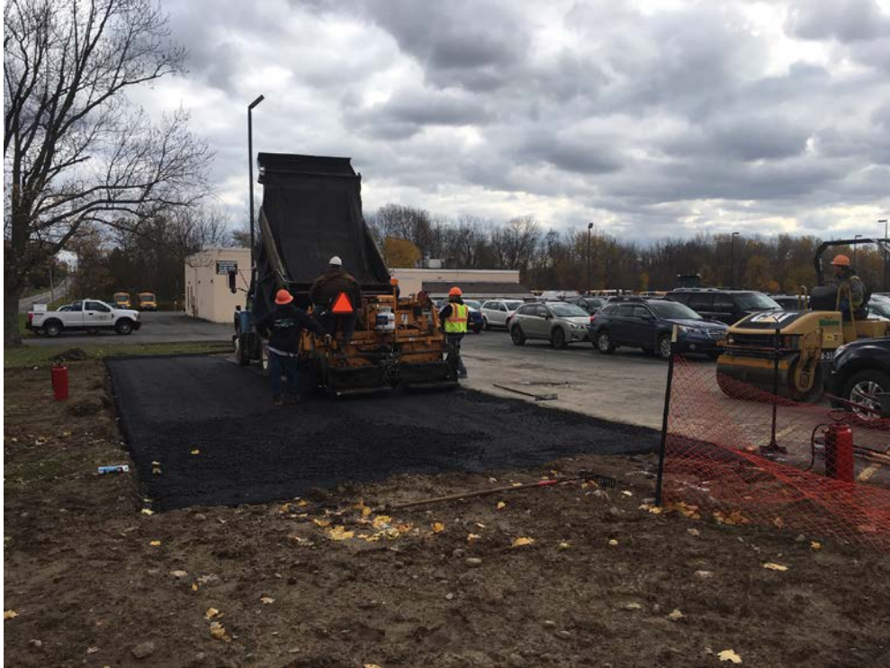
Paving of seven additional parking spaces at the ES.
