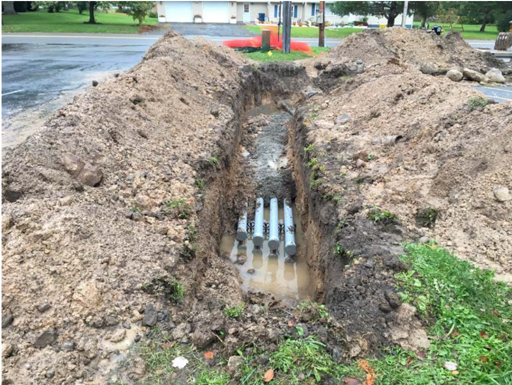
New electrical service conduit installation at the Elementary School.
