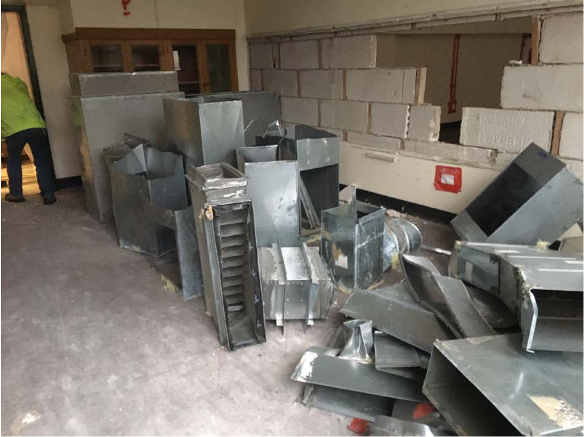
Middle School ductwork that was removed on the 2 nd floor.
