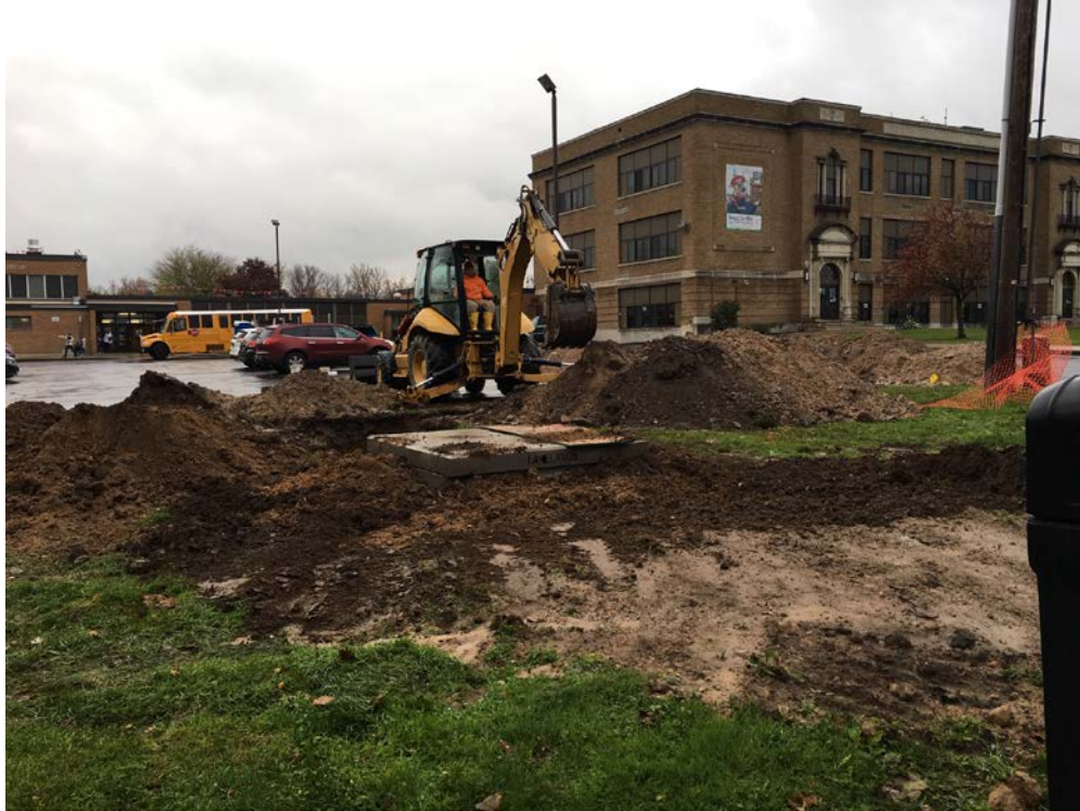
Transformer vault placement and backfilling at the ES.
